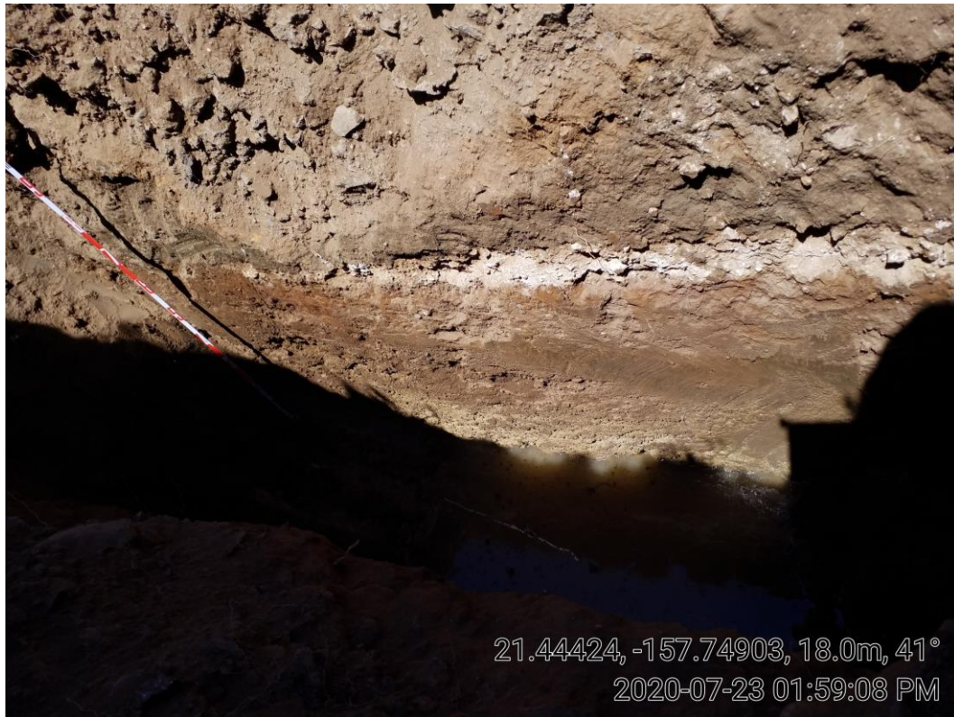
Photo 15. Trench 7, north wall profile, western end of trench.
