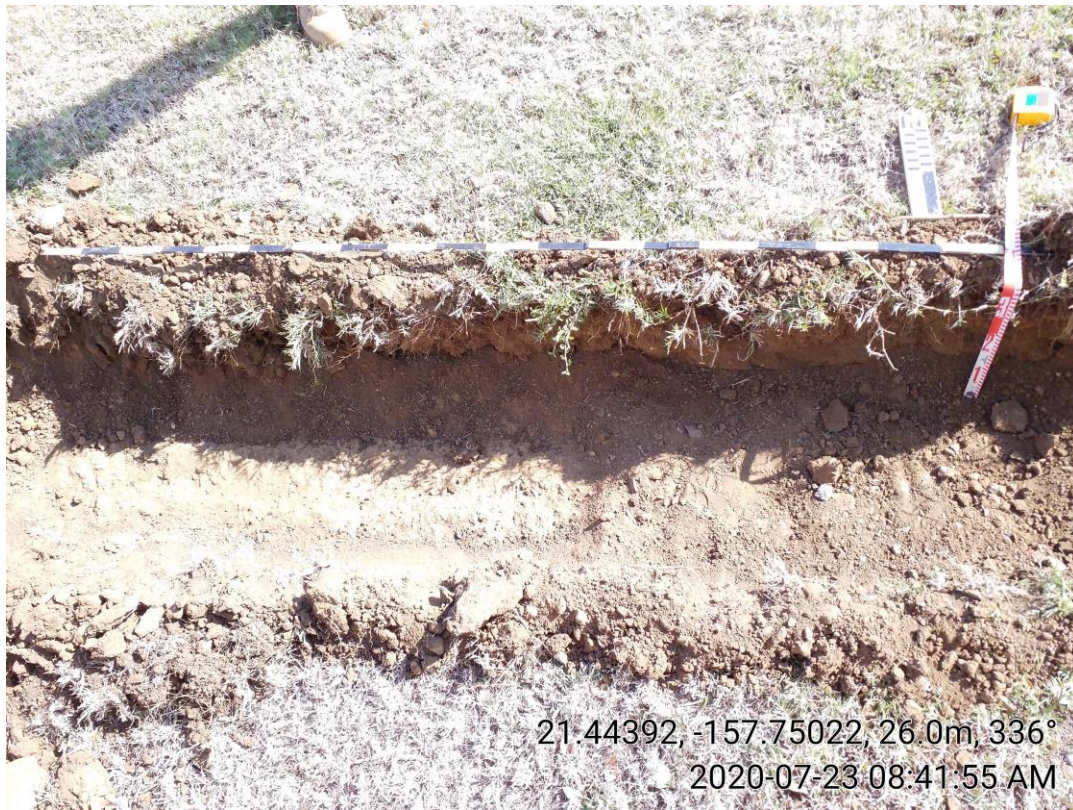
Photo 10. Trench 5a, north wall profile, center of trench.
